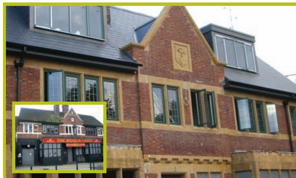
Above: The former Hand and Heart public house before (inset) and after the restoration works.
